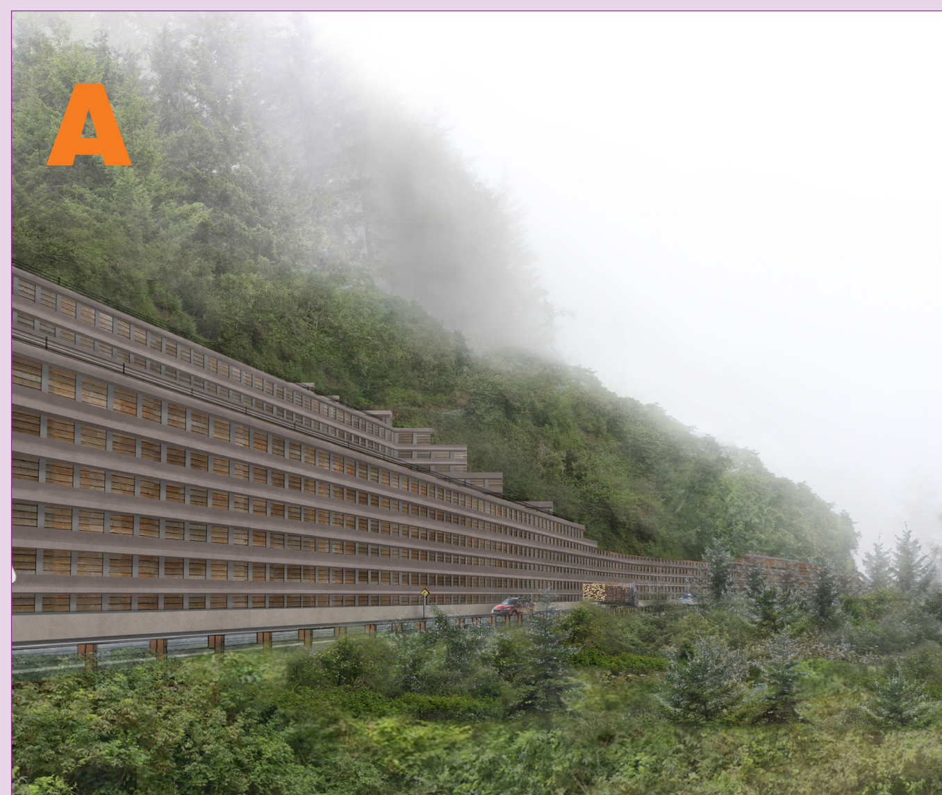
Proposed Highway Realignment and Multi-Tiered Retaining Wall viewed from Southbound U.S. 101
